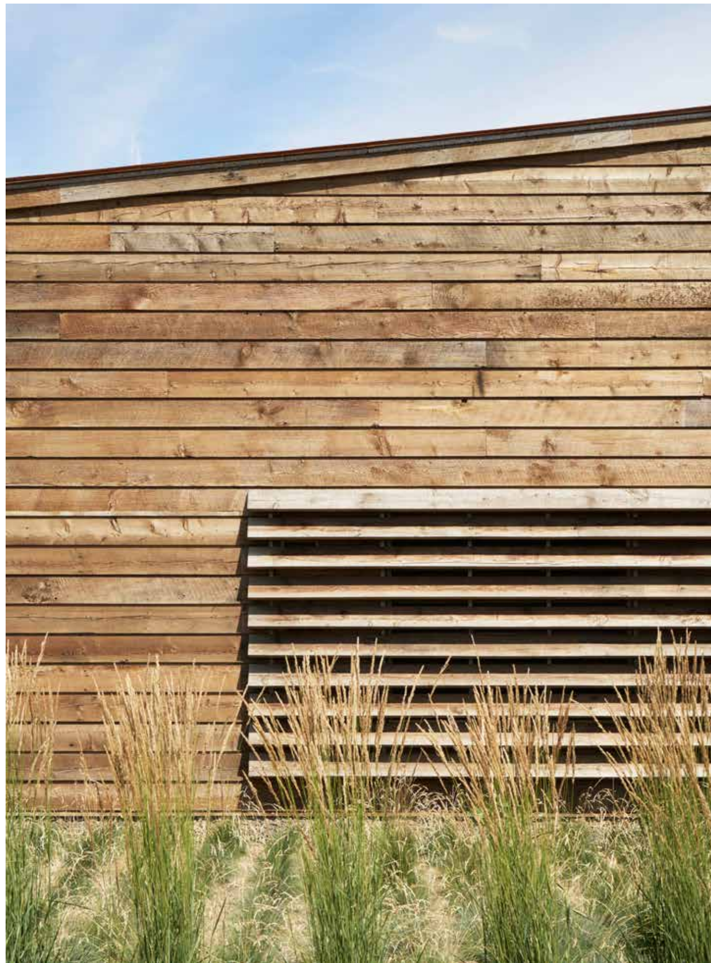
Calamagrostis and Fescue in the foreground with a backdrop of rough-sawn cedar siding and louvers.
