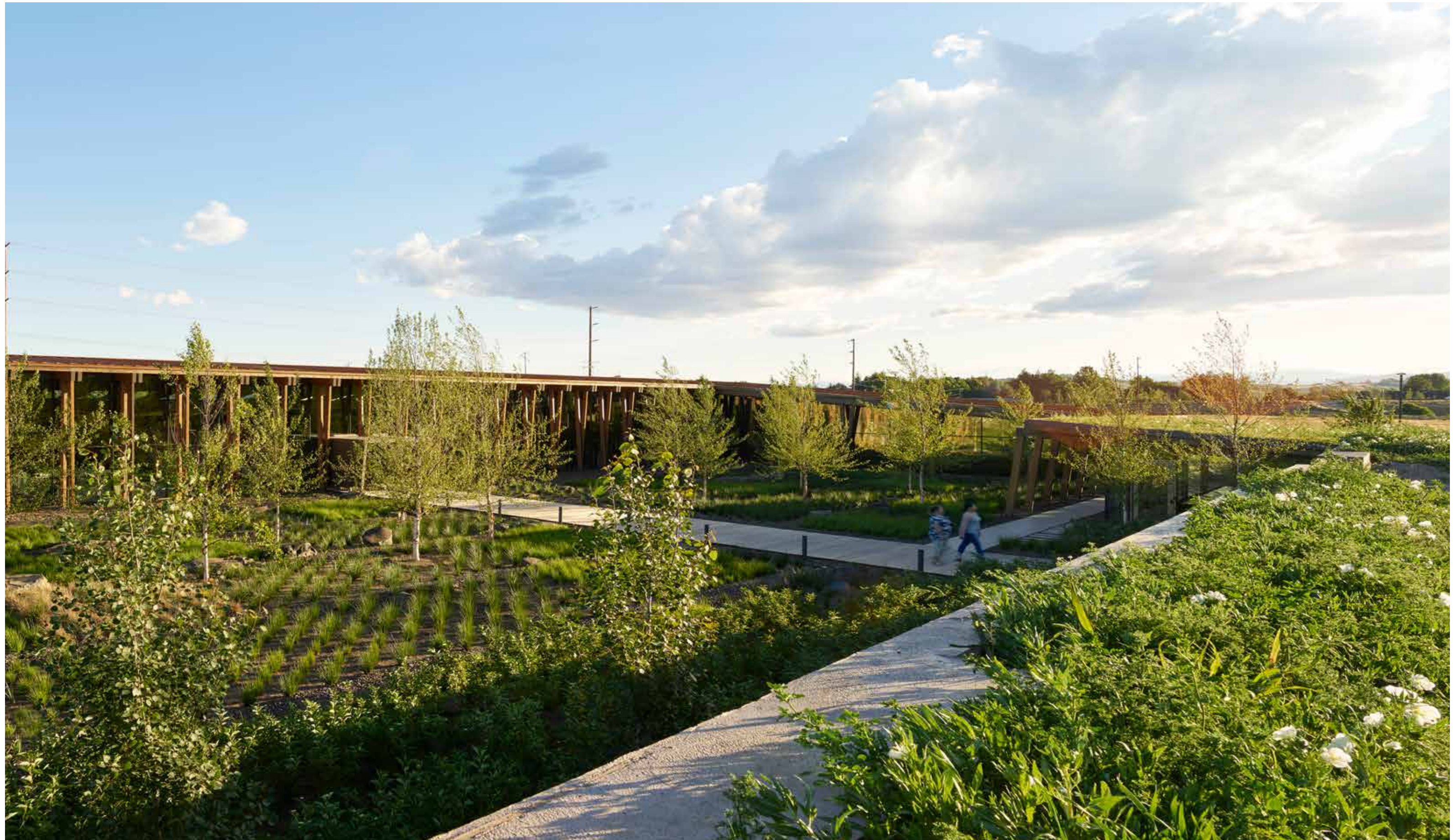
Overview of the courtyard from atop the concrete wall bisecting the northern berm. The green roof over the lunchroom is visible on the right side of the photograph.
