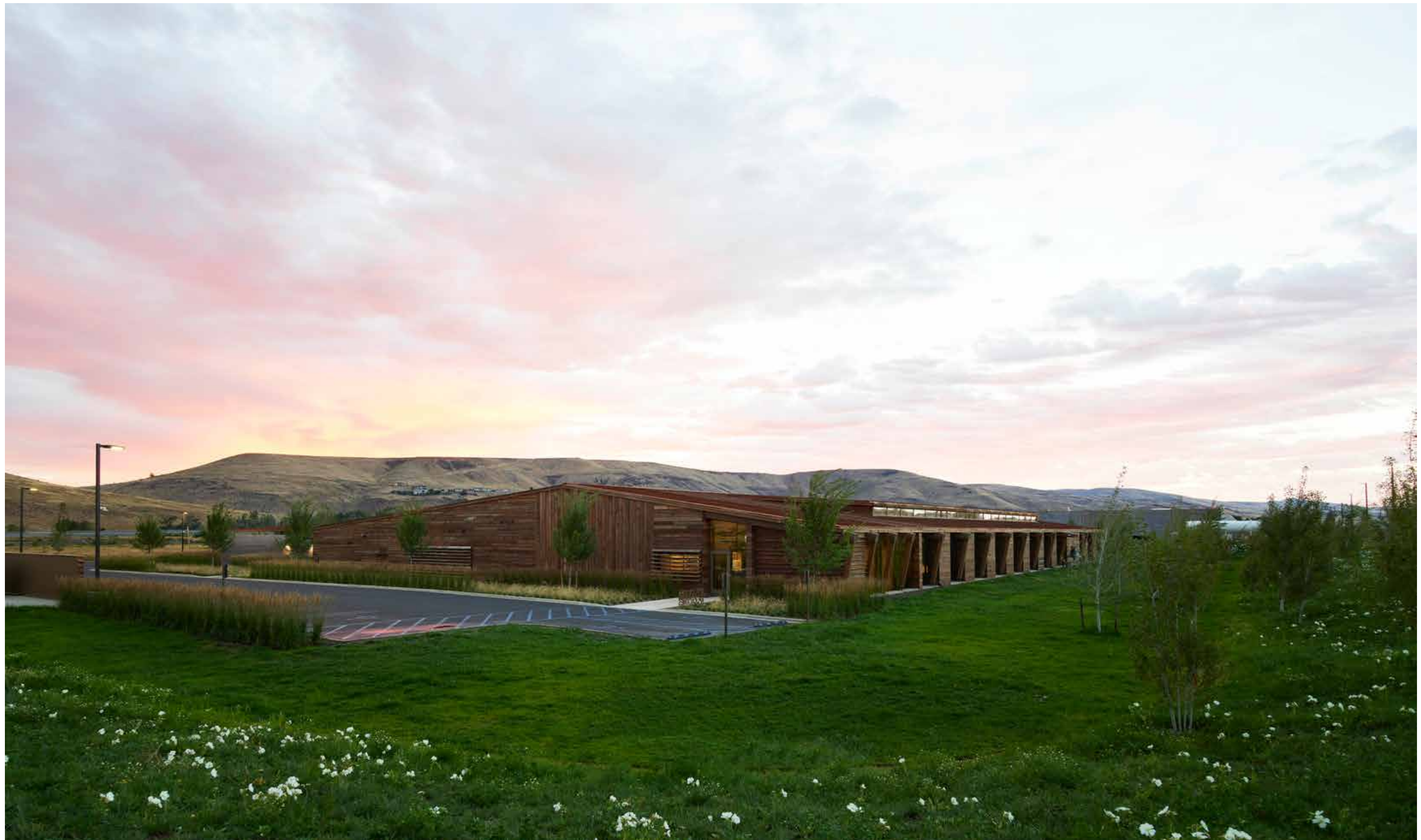
A mix of over a dozen native perennials and grasses including Evening Primrose ( Oenothera caespitosa ) blanket the mounds surrounding the office building. The lower turf area is a drought-tolerant fescue mix with reduced water and mowing requirements.
