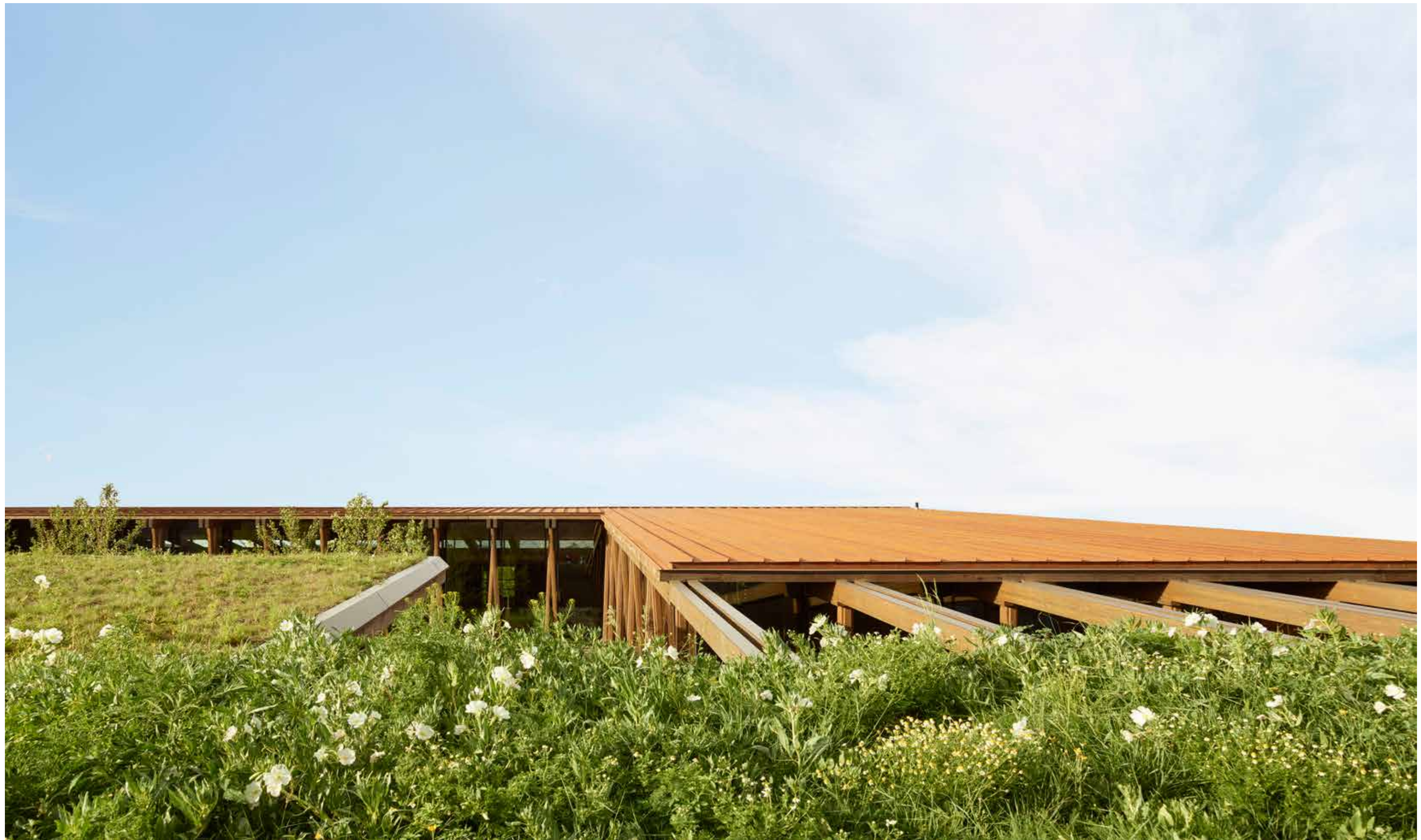
Looking south from on top of the berm illustrates the physical connection between site and structure.
