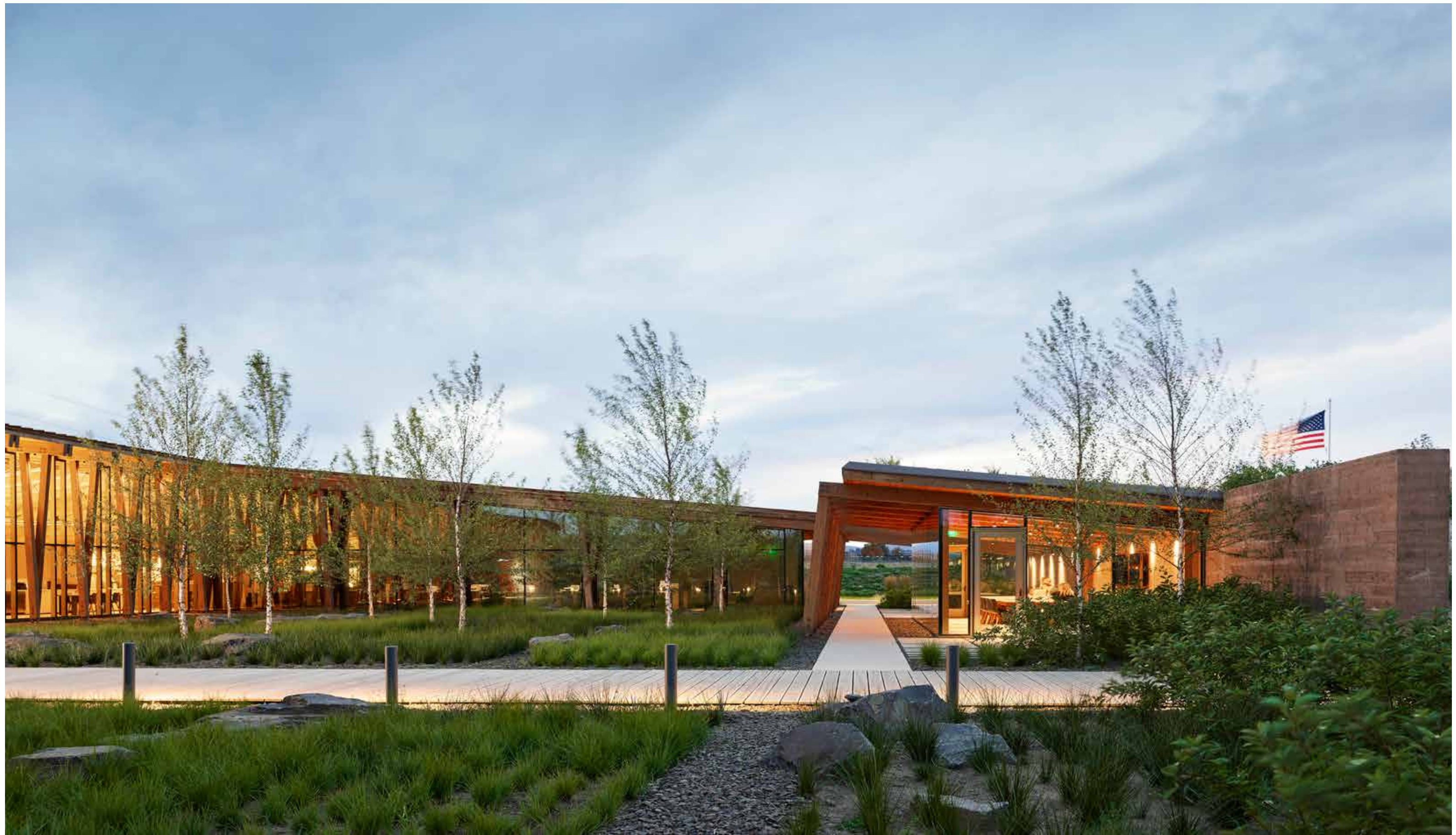
Looking west at the passage between the lunchroom and the main office, the hierarchy of paving types including wood, precast concrete pavers and crushed basalt provide intuitive wayfinding and define use.
